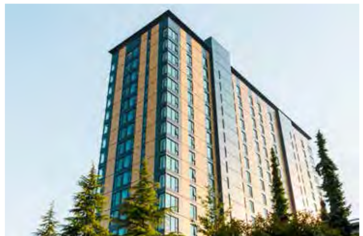
Above: Completed in 2017, Brock Commons Tallwood House is an 18 storey student residence building at the University of British Columbia. Photo: Brudner
