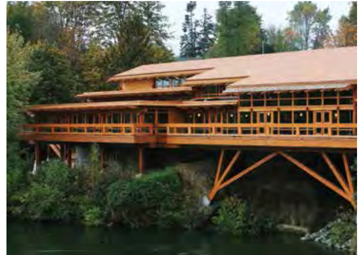
Completed October 2007, the Tseshaht Tribal Multiplex and Health Centre has a gross area of 140 m 2 (1520 ft 2 ). Photo: Lubor Trubka Architects
